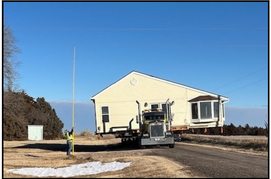
Journeyman lineman Randy Propp lifts a powerline as the oversized load travels through the district to relocate a home.
