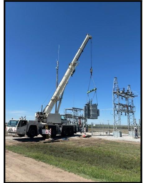
Crews upgrade the power transformer at Trenton Substation to increase capacity and cover new load growth.
