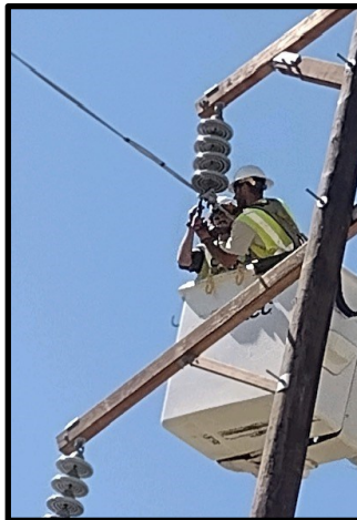
Two MPPD apprentice lineworkers hang line on a transmission structure that went down during the storm.
