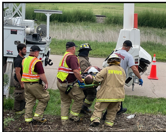
First responders transport Journeyman lineman Skyler Kalinski to level ground and prepare to load him into an ambulance.
